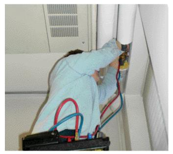
A TAB technician measuring water flow through a circuit setter.
