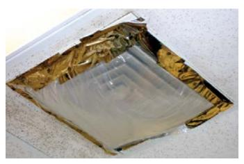
An operational issue identified during the Assessment phase, an occupant-installed damper on diffuser serving office that was too cold.
