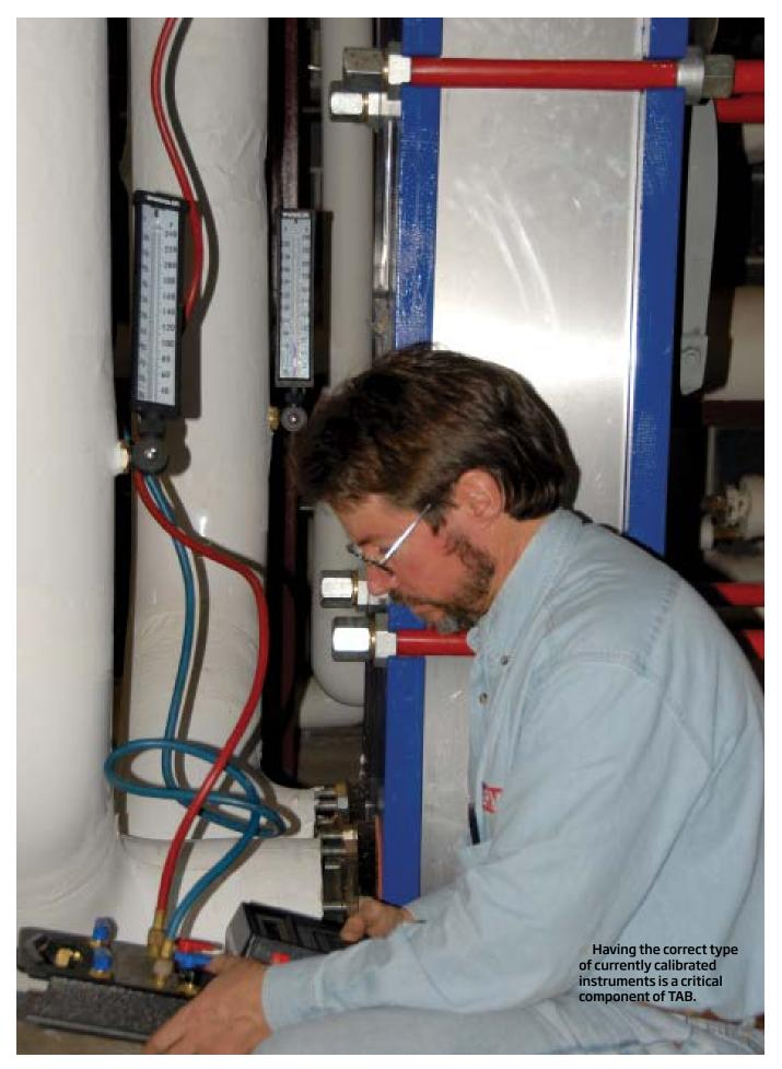
The best instrumentation in the world, used incorrectly, will yield incorrect readings. It is critically important to use instruments correctly and maintain calibration to obtain accurate and repeatable results.
