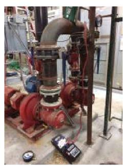
« A hydronic differential pressure meter is used to measure the actual pump or system head.
